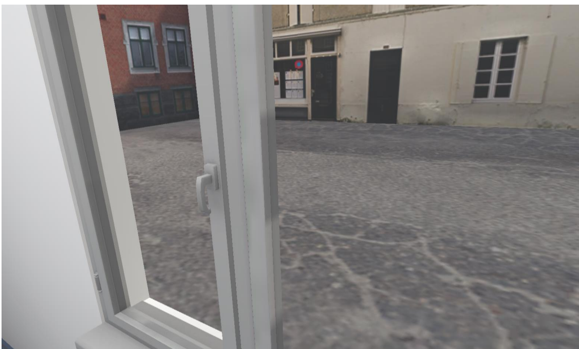
Figure 5: window with window-handle not secured against unauthorised opening
